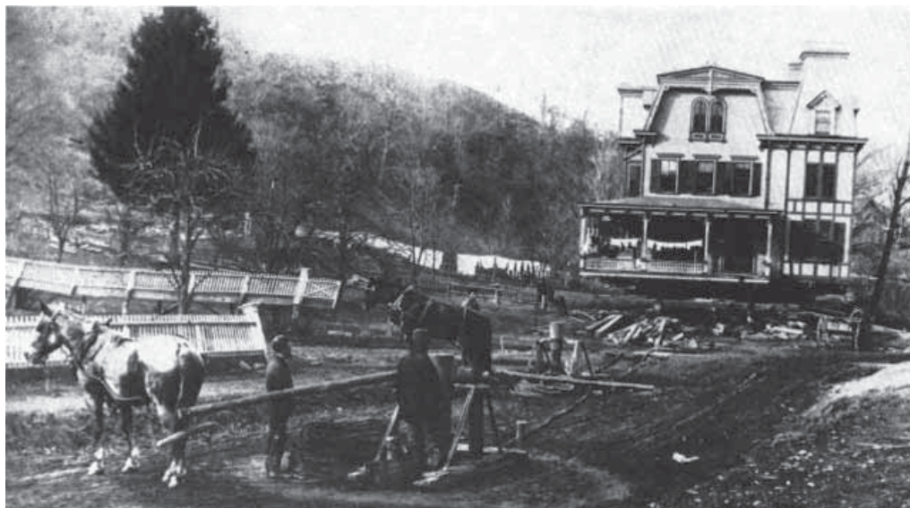
Horse on capstan uses strength and leverage to roll a house over timbers down the road
