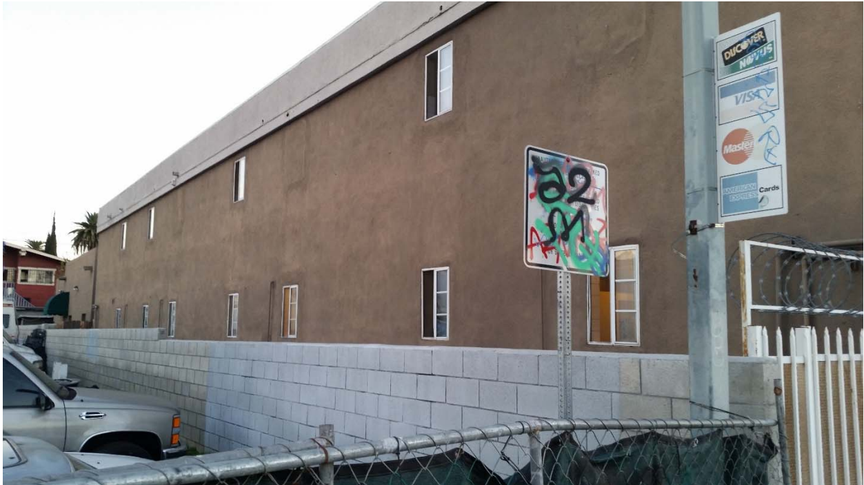
Bedroom Windows: Multiple open bedroom windows overlook the site at the fence line.
