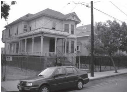
Another gutted landmark: 1978 Estrella, HCM No. 498
