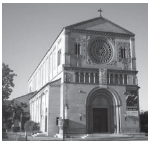
No. 516 Saint John's Episcopal Church (above) 510 W. Adams Blvd. Declared 1/22/1991
