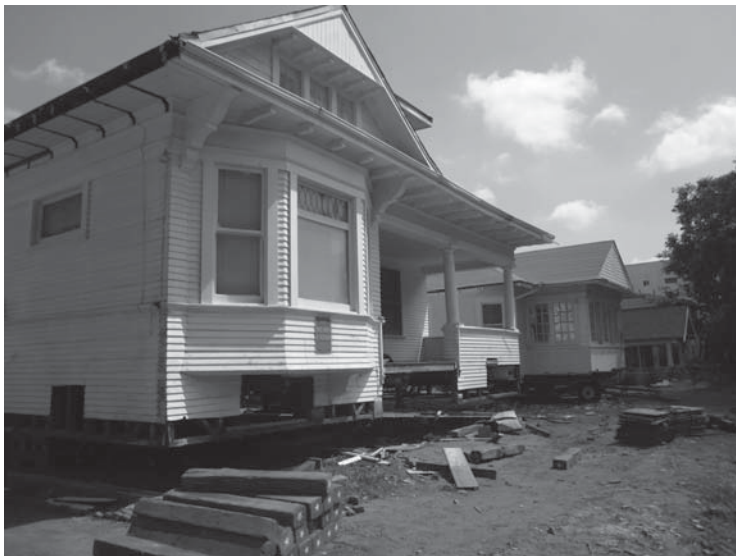
Houses up on blocks awaiting the moving truck.
