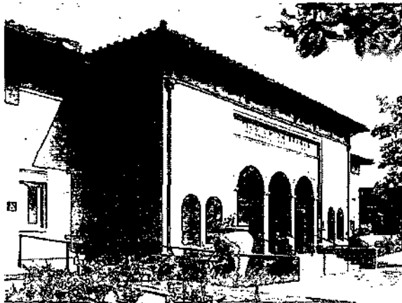
Architect Tom Michali restored the Pico Union branch library
