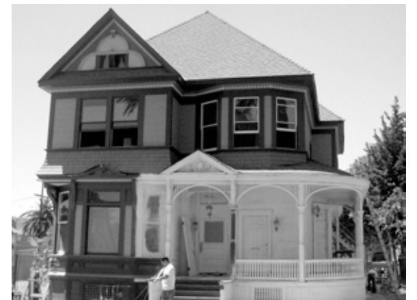
The Burkhalter Residence, after the fire (above), and in May 2009. Photos by Jim Childs (above, burned) and Jeff Valdez (below, today)
